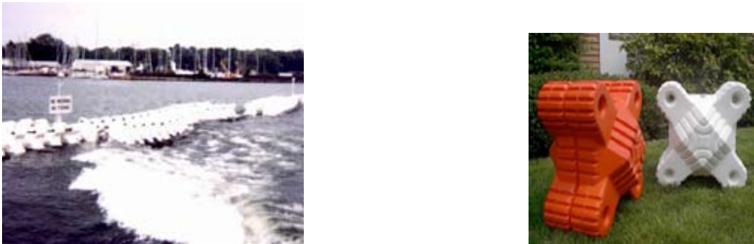
Figure 2. Floating Breakwater System (left) Consisting of an Array of Modules (right)
